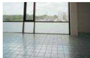
Completed Soluflex installation
